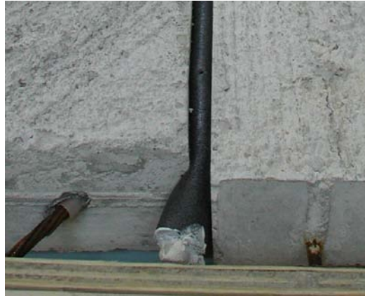
Figure 3.11 – Backer Rod between Adjacent Panels of Specimen P30P3
