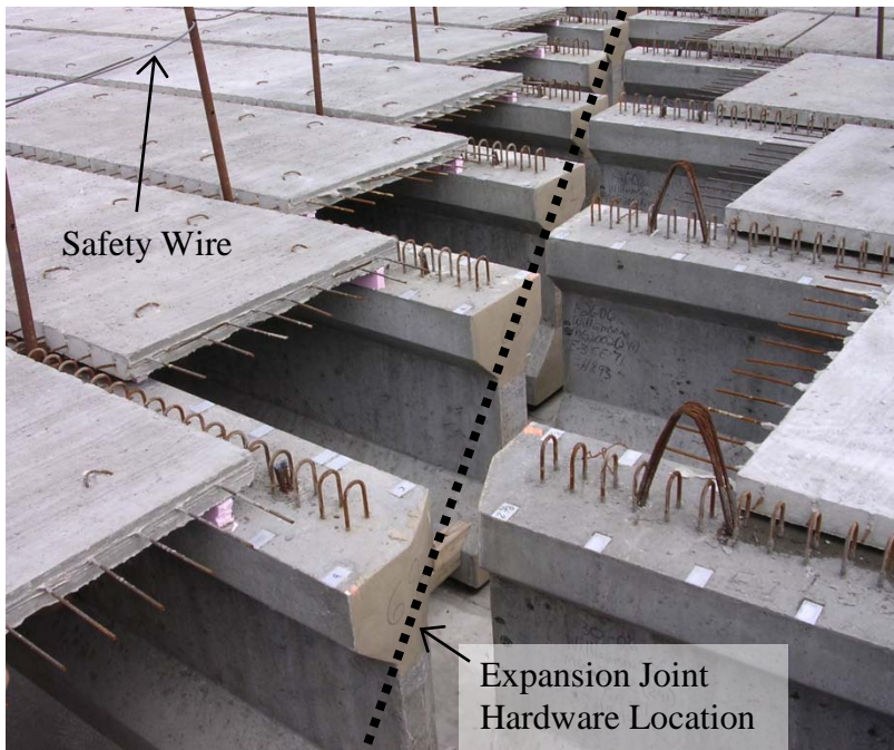
Figure 1.6: Complex Geometry and Hazardous Work Environment at a Skewed Expansion Joint under Construction (Agnew 2007)
