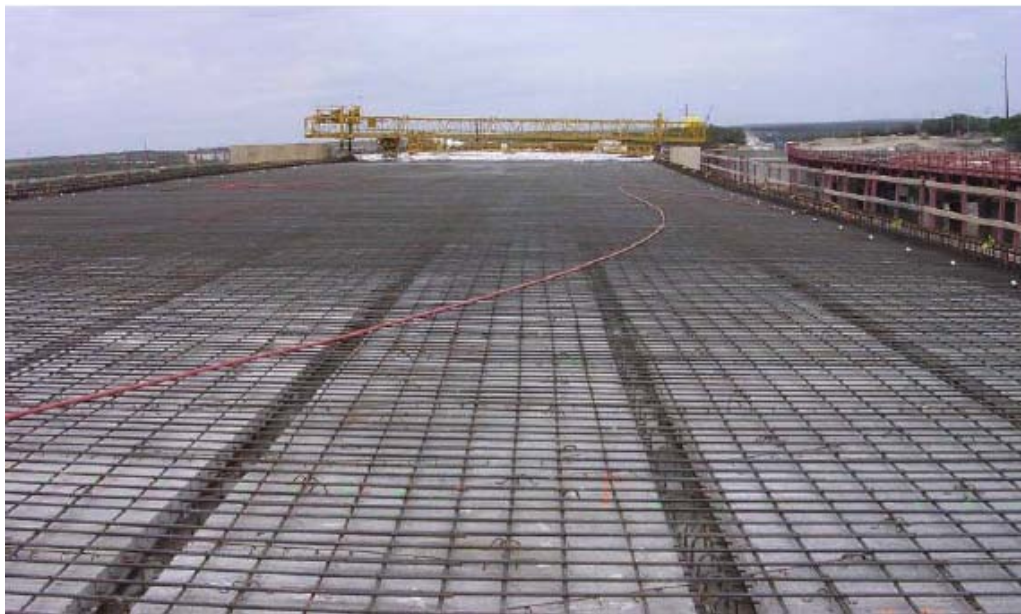
Figure 1.3: Panels and Topping Slab Reinforcement Prior to Casting Topping Slab (Agnew 2007)
